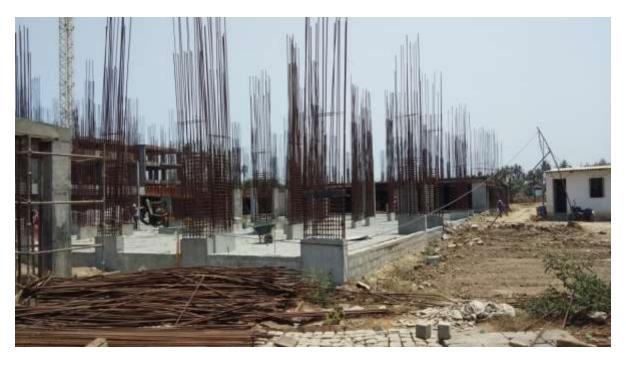
In Block D1: Excavation, Bar bending & Shuttering for Pile cap work on Progress.
