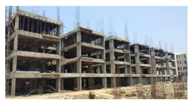
In Block B2: Pile Cap Shuttering & Bar Bending in progress..
