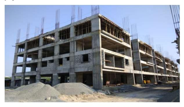
In Block C2: Second Floor level Slab 1<sup>st</sup> half Shuttering & Bar bending work in progress.
