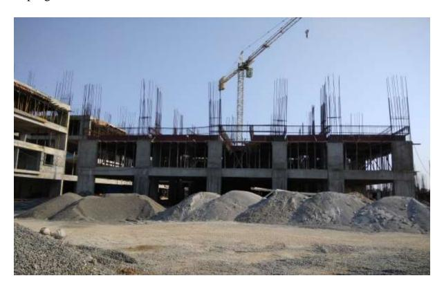
In Block C3: First Floor level Slab 1<sup>st</sup> half Shuttering & Bar Bending Work on progress.
