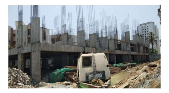
In Community Hall: Excavation, Pile cap Concrete casting, pile chipping &Column Casing work on progress.
