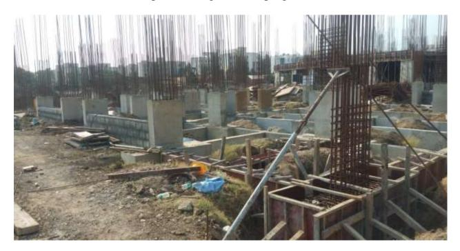
In Block A2: Pile Cap Plinth Barbending work on progress.
