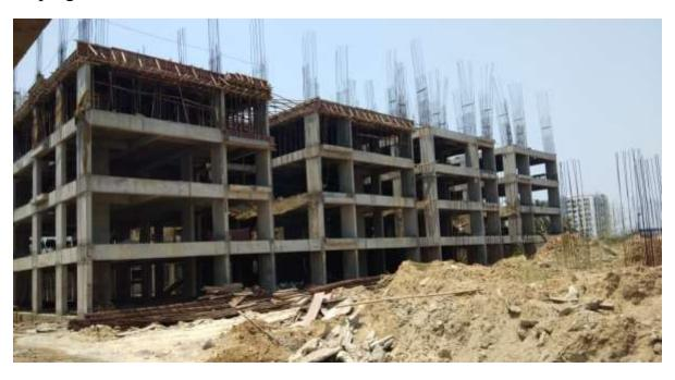
In Block D3: First floor Column Shuttering and Bar bending Works in Progress.
